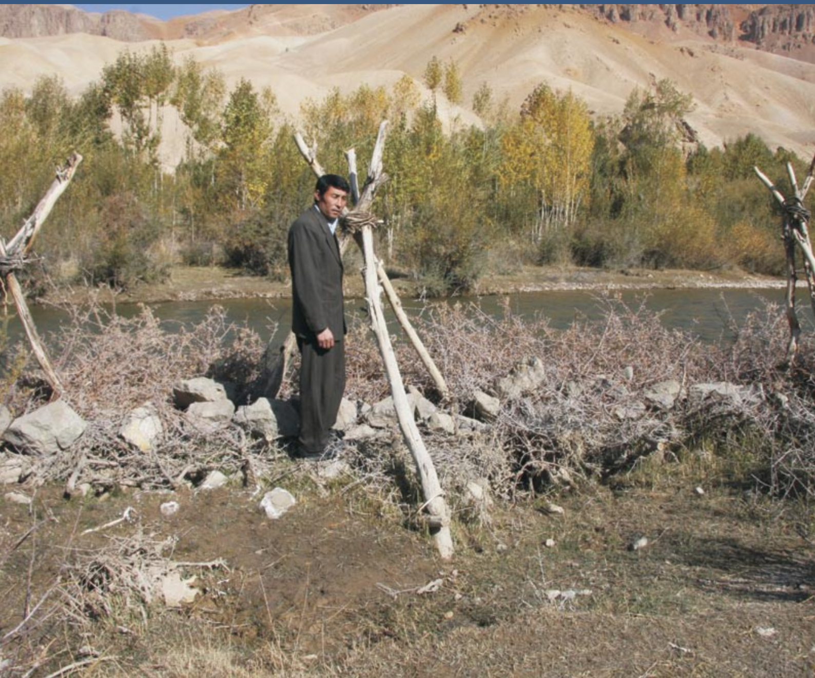
Using local indigenous technologies, known as Daka, to stabilize river banks at a UNEP CBNRM site in Yawkalang, Bamiyan.
